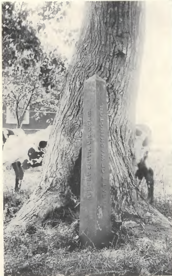
ONE OF THE OLD SMITH-ESTCOURT MONUMENTS ON THE QUEBEC-VERMONT BOUNDARY. ORIGINALLY IN THE CLEAR IN 1845 IT HAD TO BE MOVED AFTER THE TREE HAD GROWN.
