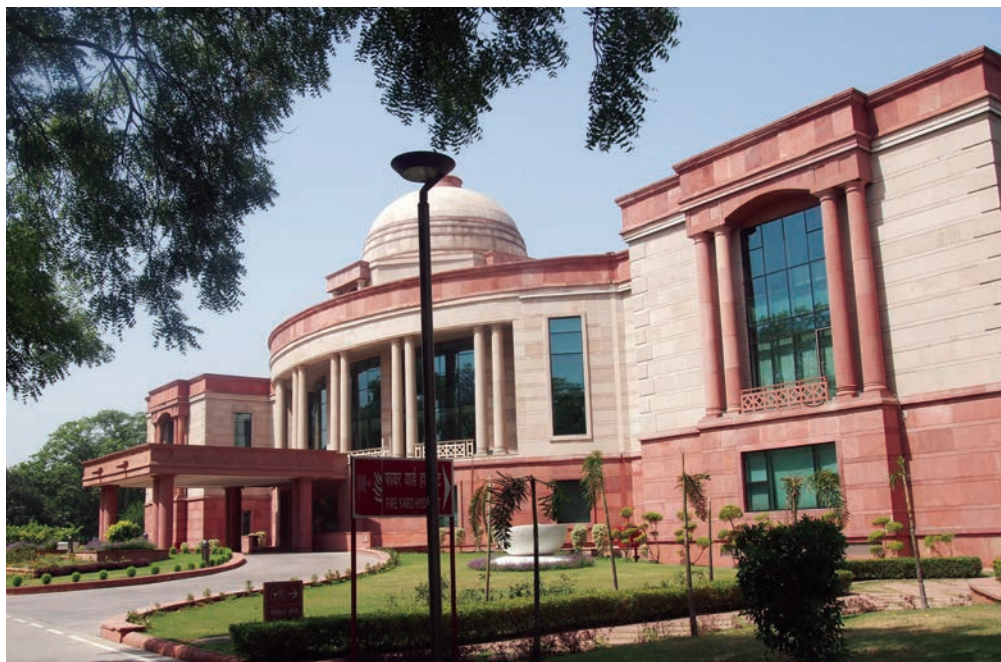
Jawaharlal Nehru Bhavan is the new home of India's Ministry of External Affairs. The red sandstone structure with a built-up area of nearly 60,000 square meters is state-of-the-art and has many green features. It is the first government building that is compliant with the country's 2007 Energy Conservation Building Code and is LEED-certified.
