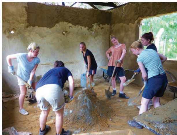
On a typical day at one campsite, gap-year students help with construction work in a village.
