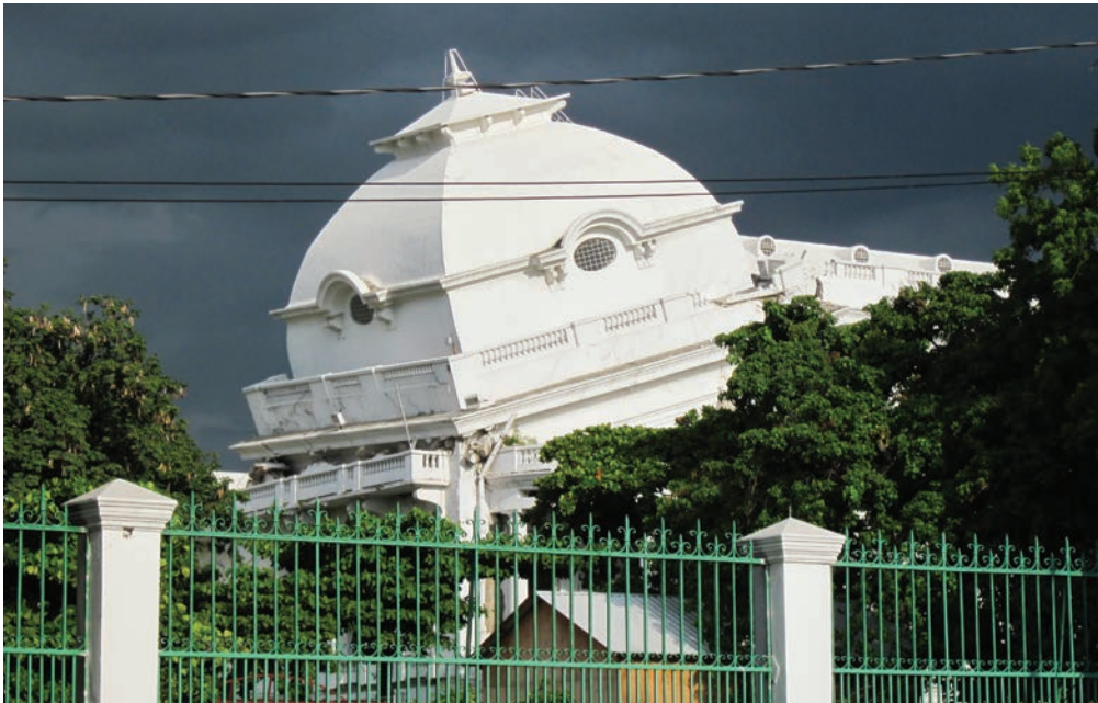
One wing of the Presidential Palace in downtown Port-au-Prince collapsed during the January 2010 earthquake.
