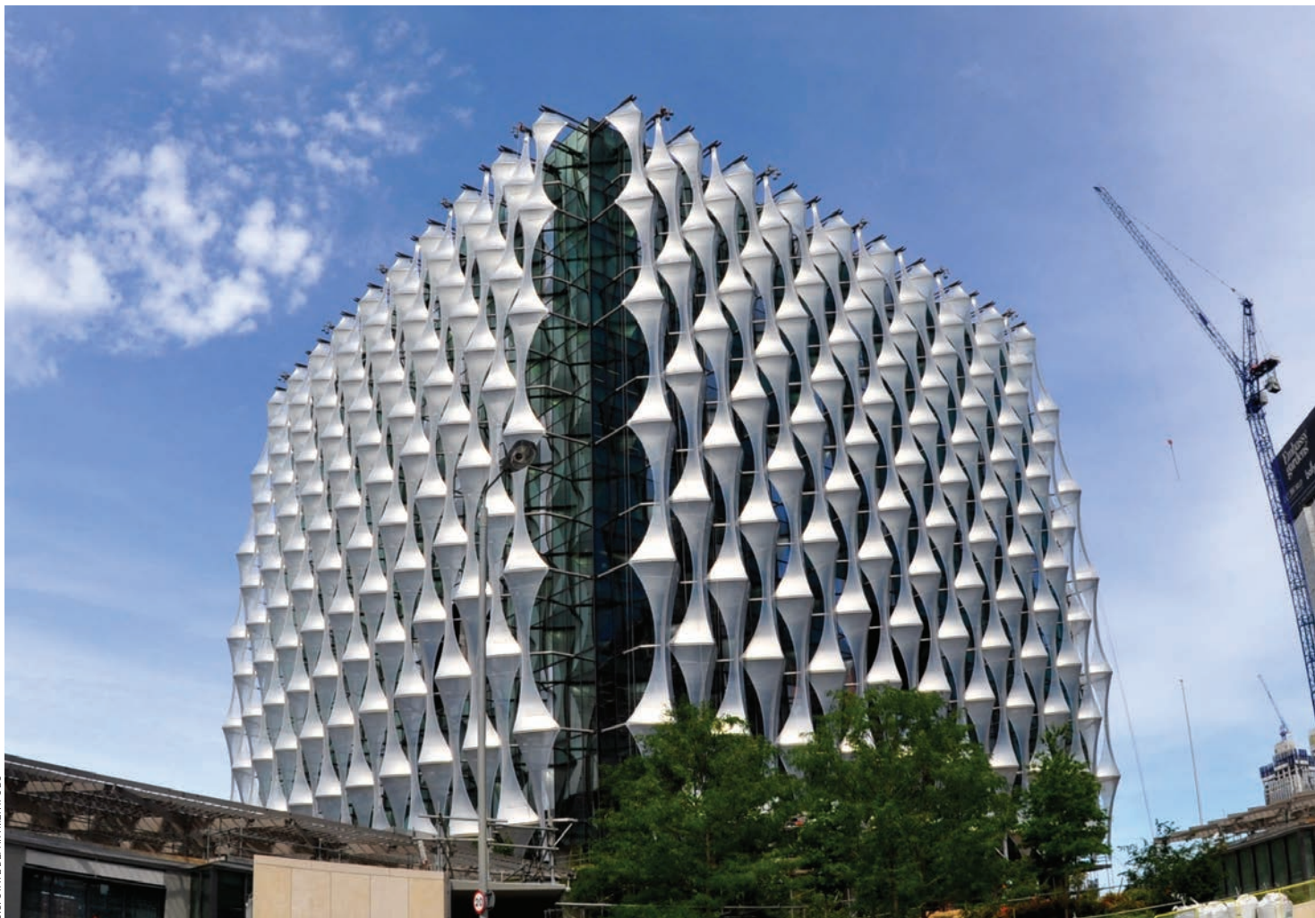
The new U.S. Embassy London up close. The lightweight plastic scrim that give a soft and billowy look to the exterior are embedded with photovoltaic cells that can convert sunlight into energy. At the same time, they will act as sunscreens to keep interiors from overheating.
