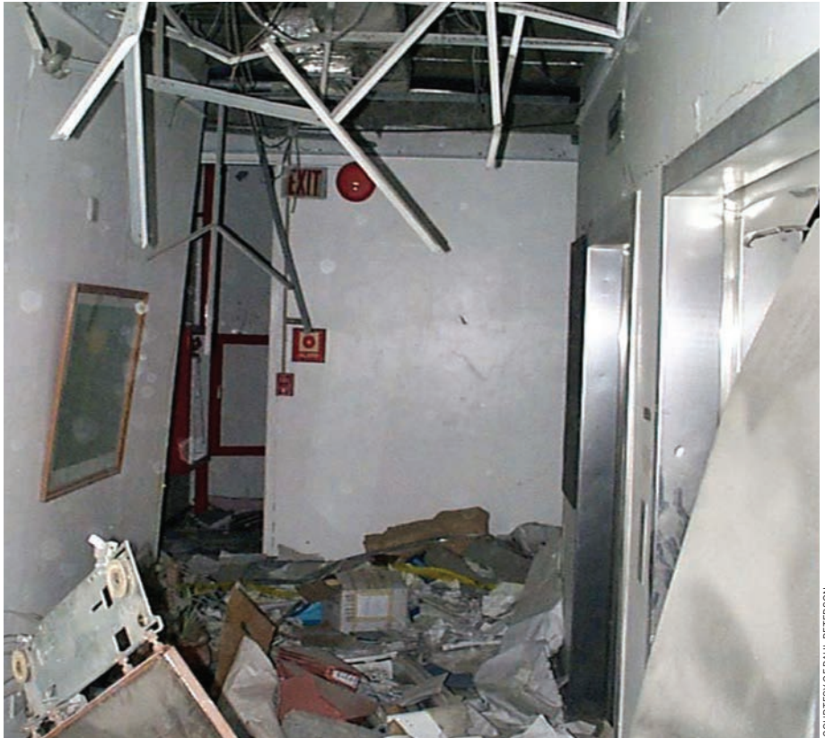
Elevators in U.S. Embassy Nairobi were destroyed in the blast. A woman was rescued by first responders from under the debris at this spot.
