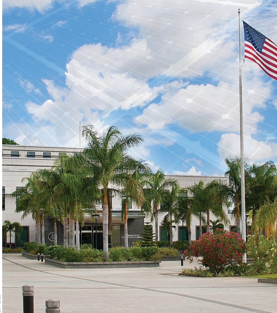
Embassy Managua will reduce energy purchased from the grid by 54 percent through an Energy Saving Performance Contract with Lockheed Martin to install a 1-MW photovoltaic array, replace interior and exterior lighting with LED illumination and improve the chiller equipment.
