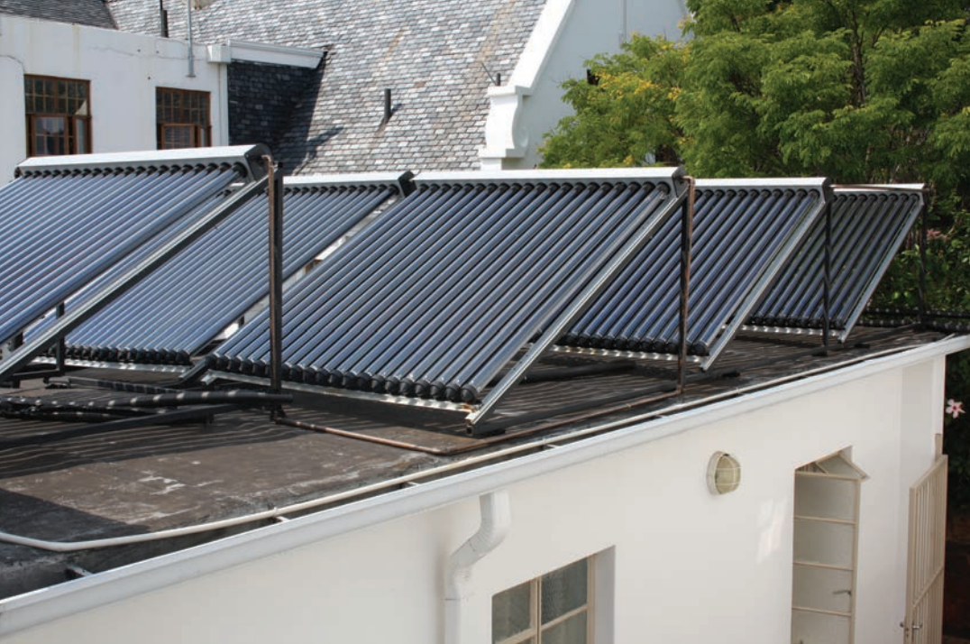
This solar hot water recirculation system installed on the ambassador's residence in Pretoria replaced 10 electric water heaters.
