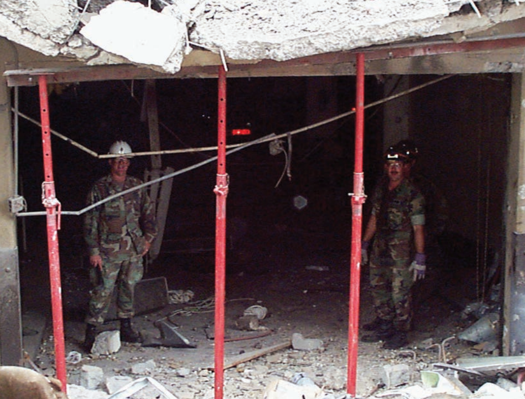
Navy Seabees shoring up damage to the underground parking area at the embassy in Nairobi.
