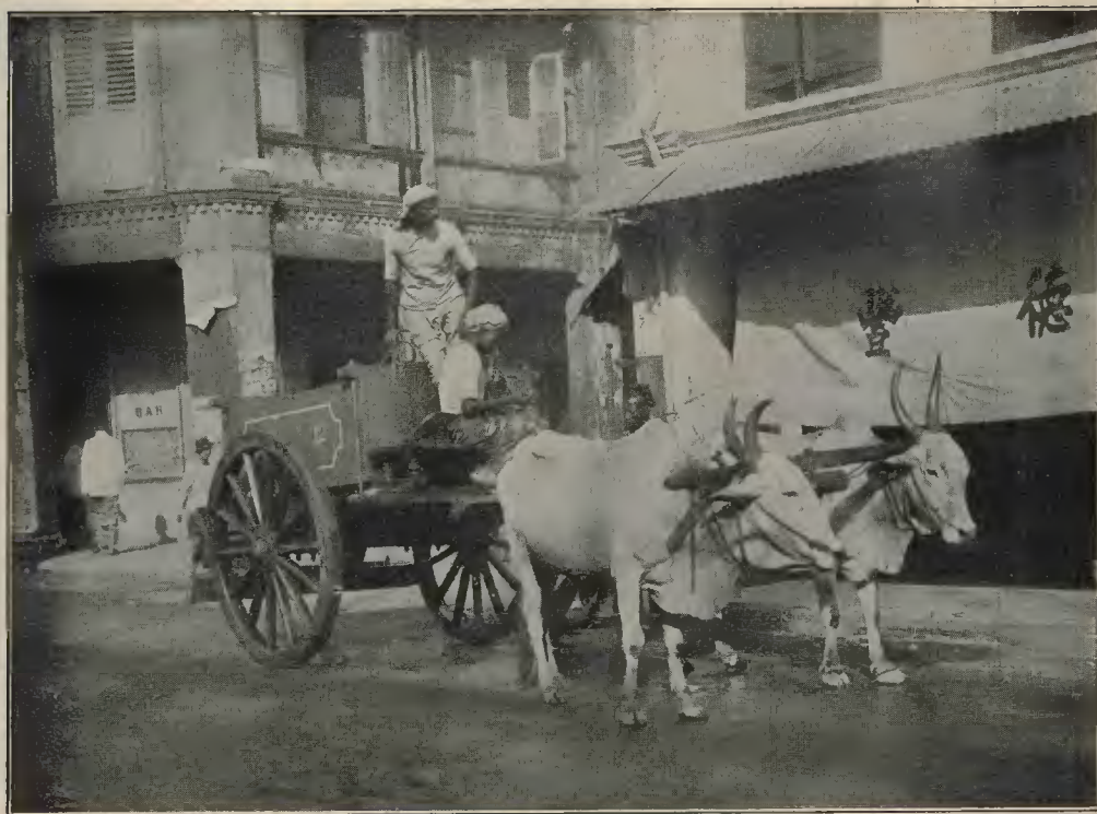
A SPRINKLER IN SINGAPORE
