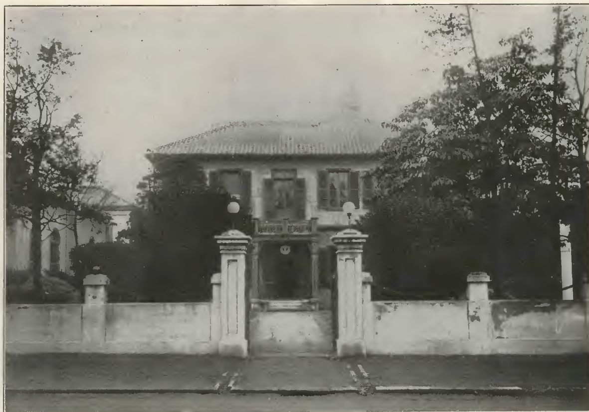
AMERICAN CONSULATE GENERAL AT YOKOHAMA The building collapsed during the earthquake on September 1, 1923
