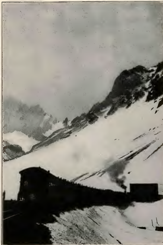
Entering the tunnel which crosses the Chile-Argentine frontier. The view is taken at Caracoles, Chile, and the continental divide can be seen in the distance at the left
