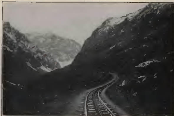
Rack, or cogwheel railroad, used on the steep grades of the Transandino. Three cogwheel drivers of the locomotive fit into the three racks laid midway between the rails
