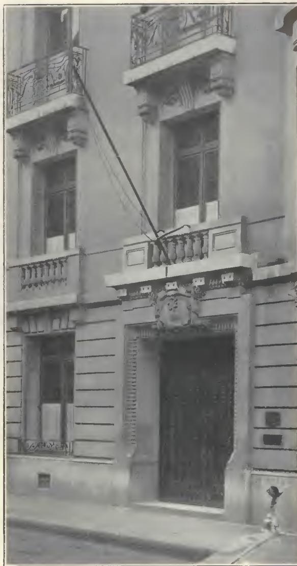
ENTRANCE TO THE PASSPORT OFFICE AT PARIS
