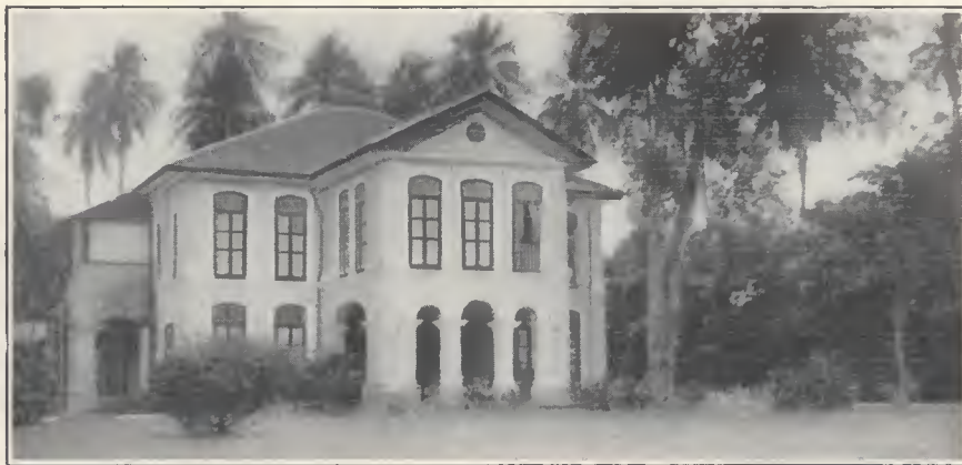
CONSULATE AND RESIDENCE AT PENANG
