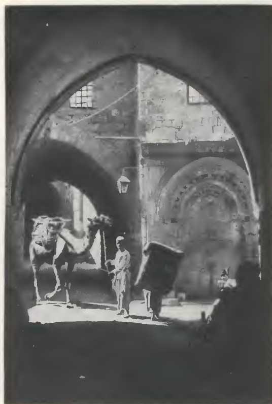
Photograph by Mzyard Owen Williams.
