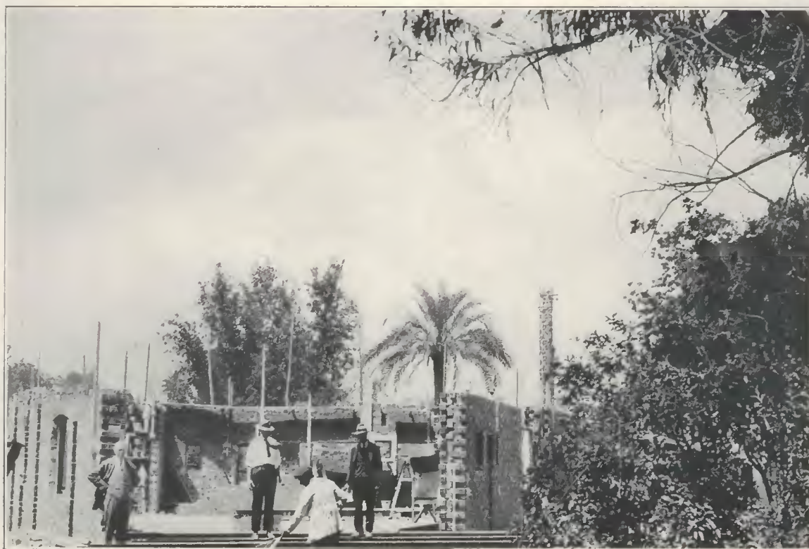
CONSTRUCTION WORK ON MAY 20, 1928
