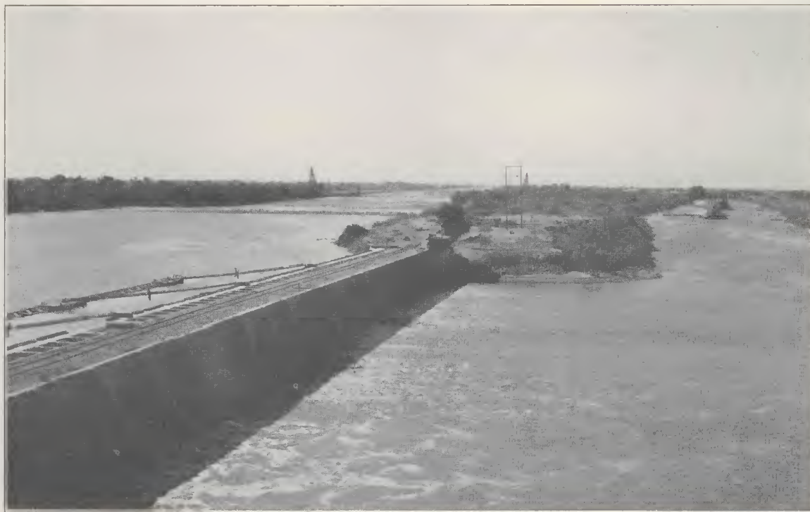
ROCKWOOD IRRIGATION INTAKE GATES
