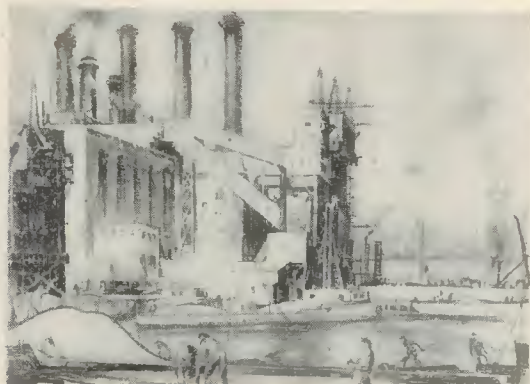
The Power Plant
