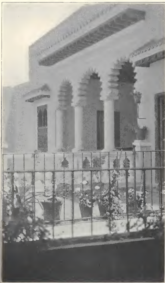
Photo from Honor M. Bigelow UPPER PORTION OF NEW WING OF AMERICAN LEGATION, TANGIER, COMPLETED IN 1931
