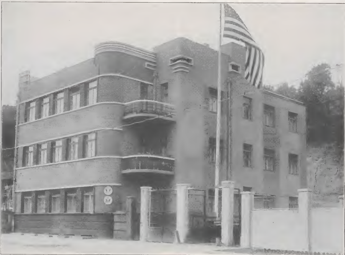
THE NEW LEGATION-CONSULATE AT KAUNAS (Occupied November 4, 1930)
