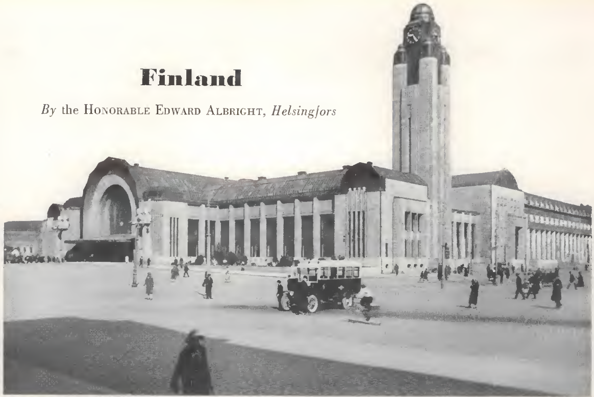
RAILWAY STATION, HELSINGFORS, DESIGNED BY ELIEL SAARINEN
