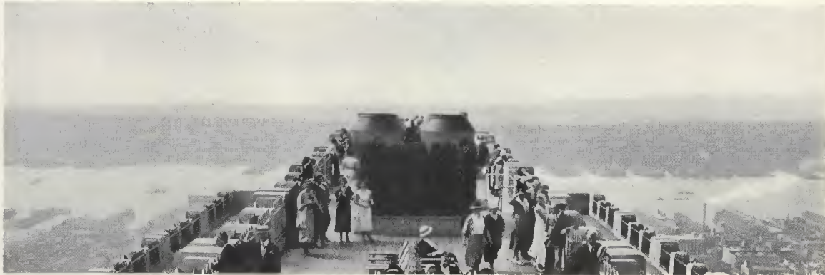
OBSERVATION ROOF OF THE 70-STORY R C A BUILDING
