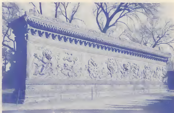
THE DRAGON SCREEN IN THE WINTER PALACE GROUNDS, PEIPING
