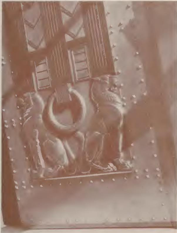
PART OF THE MASSIVE ALUMINUM ENTRANCE, TWENTY-FIVE FEET HIGH, WHICH STANDS AT THE PORTALS OF THE NEW DEPARTMENT OF JUSTICE
