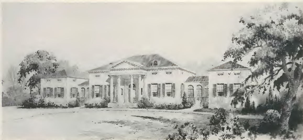
THE NEW AMERICAN LEGATION-CONSULATE GENERAL, MONROVIA
