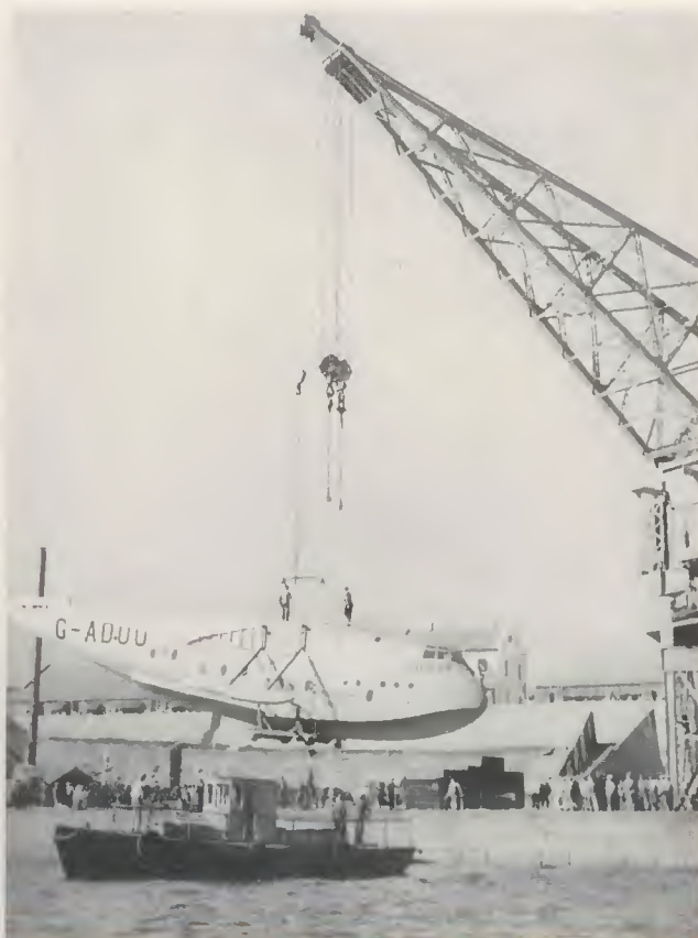
UNLOADING THE HULL OF THE "CAVALIER" AT HAMILTON
