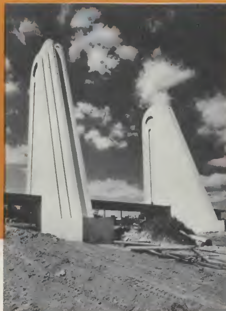
Two entrance pylons
