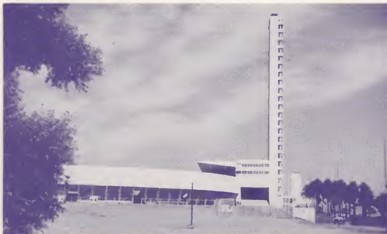
Helsinki Olympic Stadium, showing the tower and a section of the grandstand.
