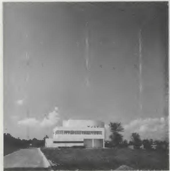
WJSV, Columbia Broadcasting Company, fifty-thousand watt transmitter at Wheaton, Maryland.
