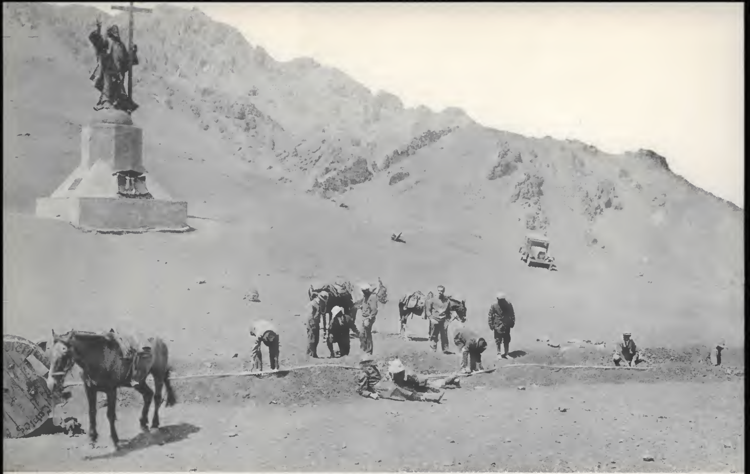
At the feet of CHRIST OF THE ANDES, world famous monument to eternal peace between Chile and Argentina, engineers of the I. T. & T. Corp. bury the transcontinental circuits that enable the peoples of the opposite shores of South America to talk with each other.
