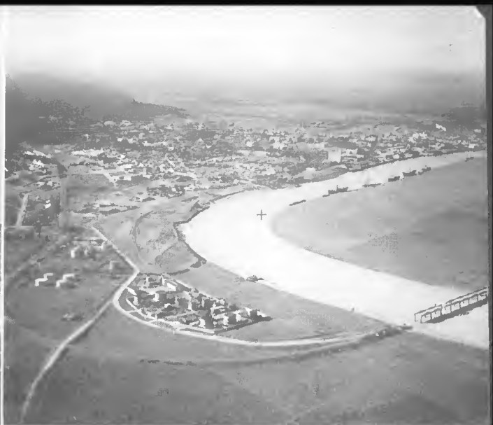
Port Lyautey, French Morocco. Damaged bridge northeast of Port Lyautey, north of Casablanca.
