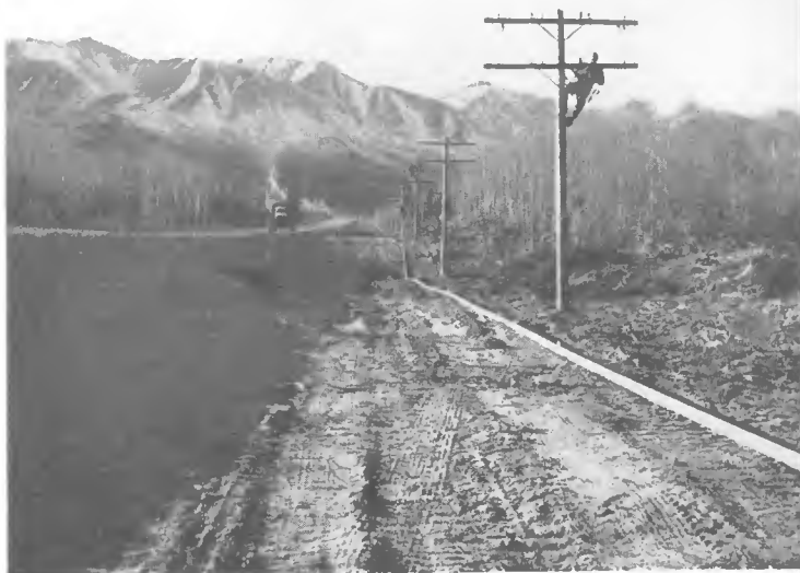
Stretch of the Highway showing pipeline and telephone line.
