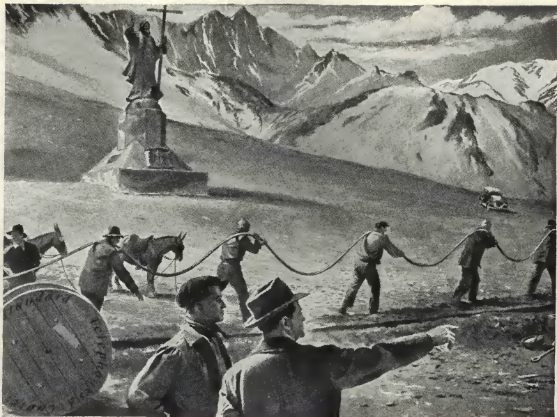
Laying the great telephone and telegraph cable of All America Cables and Radio, Inc., interconnecting Argentina and Chile, past the feet of "The Christ of the Andes" . . . 13,780 feet above sea level.
