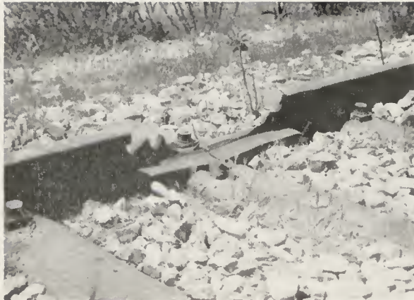
The Germans made an art of destruction, especially of railroads and bridges. The above photograph shows the work of a special rail-destroying machine which gouged out alternate rails, every few yards.
