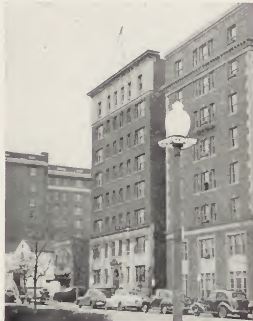
New quarters of the Foreign Service Institute in the Mayfair Building, 2115 C Street, near the new State Department headquarters.
