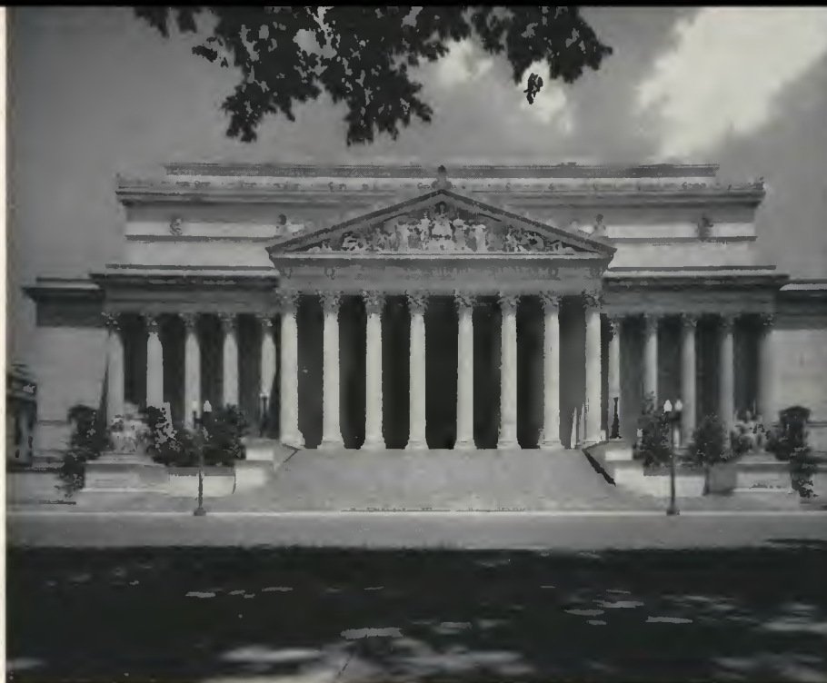
National Archives Building, Washington, D. C.
