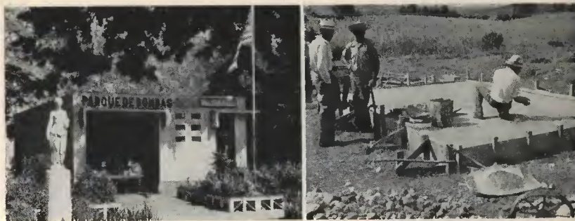
Photos by Roskam—Puerto Rico Office of Information Left: San Juan. In the foreground is a modern fire station—in the background, the old city wall. Right: The resettlement program is helping many formerly landless farmers like these build their own homes. Here the cement floor is being finished.
