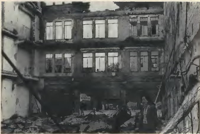
Interior of USIS Building
