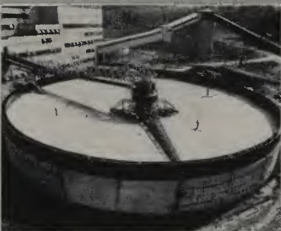
Thickener Installation
