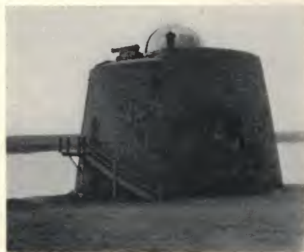
Martello towers, part of the old fortifications
