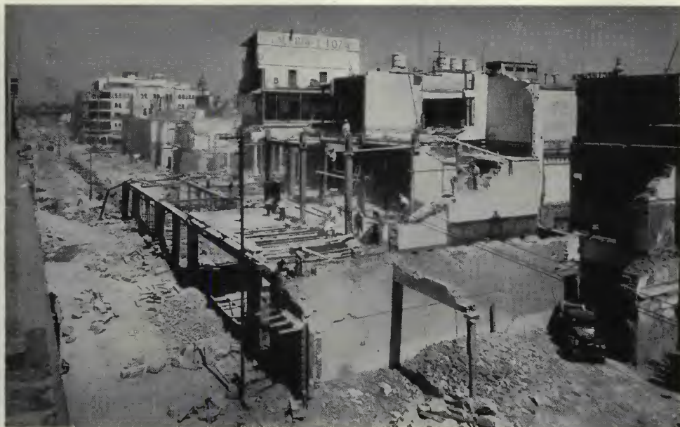
Avenida Juarez during reconstruction.
