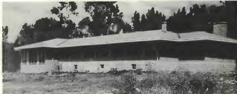
A new office building, constructed in the Embassy compound in Addis Ababa, Ethiopia.
