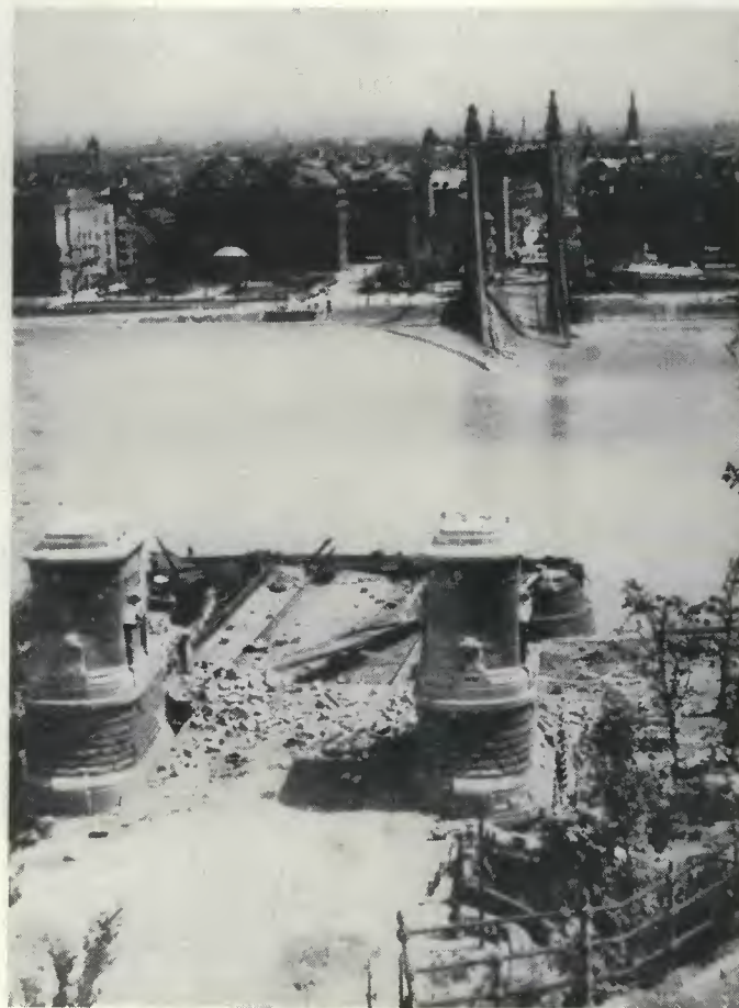
The St. Elizabeth bridge, looking from Buda.
