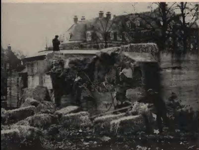
An old World War II bunker in Amsterdam is destroyed. Note the bales of straw piled over the dynamite charge in order to prevent the fragments of concrete from flying to nearby buildings.
