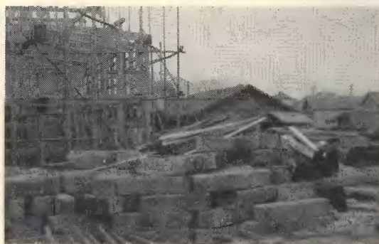
One of the old Dutch factories, now being rebuilt.
