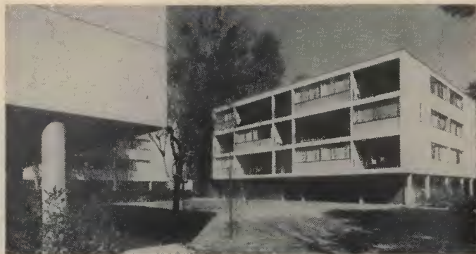
U. S. Embassy Staff Apartments at Neuilly which were given Award of Merit by the American Institute of Architects.
