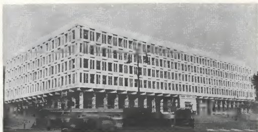
New Embassy Office Bldg., under construction in London, 1959
