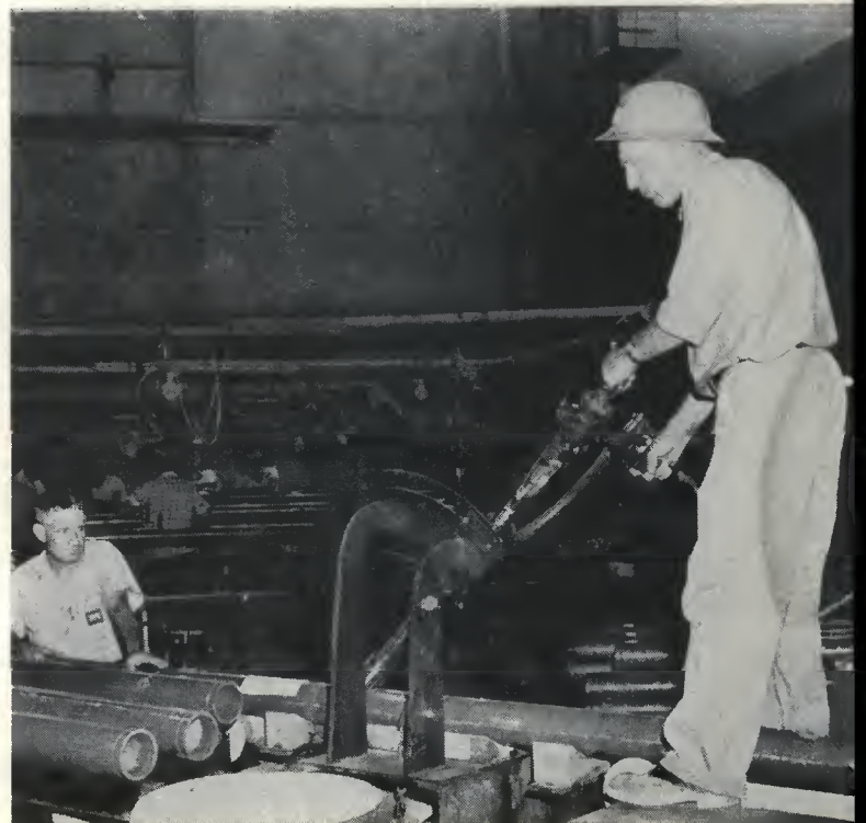
Another Kellogg team handles boring of plastic piping on a mass production basis
