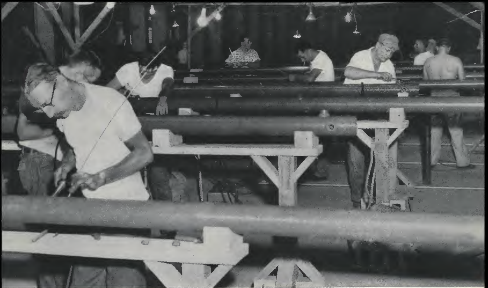
Kellogg production line at the plant site welds plastic piping to fittings
