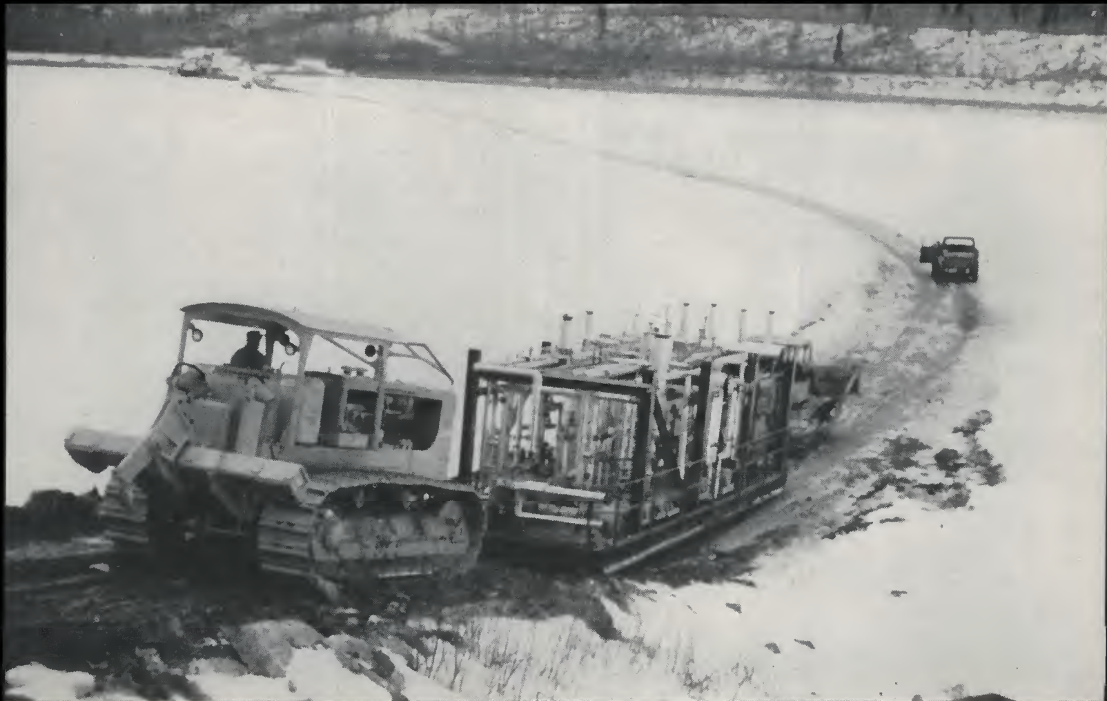
Crossing the ice bridge near Fort McMurray, the first of nine plant sections—each on self-contained runners—starts the 35-mile "skid" to the site.
