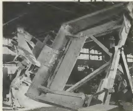
**GIANT SCRAPER'S YOKE STRUCTURE**, side sheets, body truss tubes, apron arms are of USS MANTEN\* high-strength steel; yield point at least 1½ times that of carbon steel (ASTM-A7), permitting thinner, lighter sections.
