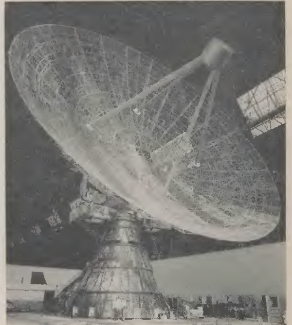
(1) BMEWS construction site at Fylingdales Moor, Yorkshire, England. Arrows point to rotating radar tracking emplacements. (2) U.S. Navy ships supplying BMEWS Thule during ice-free summer. (3) Prototype of 175-ton BMEWS rotating tracking radar at Thule and Fylingdales Moor. (4) The author in front of detection radar grid at BMEWS Thule. (5) Air view of BMEWS Thule showing tracking radar (arrow) flanked by two of four huge detection radars.
