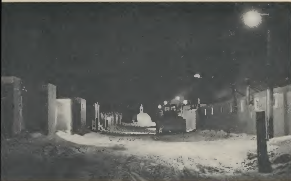
Street scene, McMurdo Station, during winter season. Buildings in immediate foreground are CPO Quarters and station galley and mess hall.
